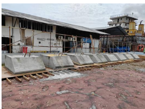
First set of eight new 5MT mooring blocks being casted.
